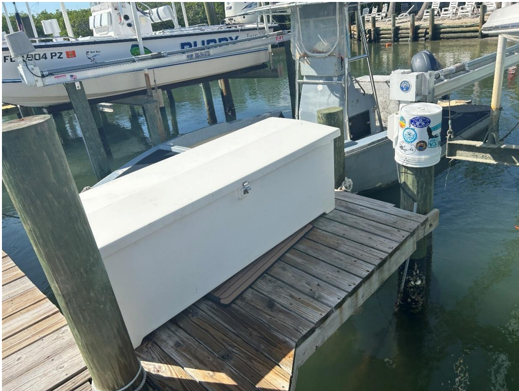
Photo 9: Small finger pier, used for deck boxes, facing southeast.
