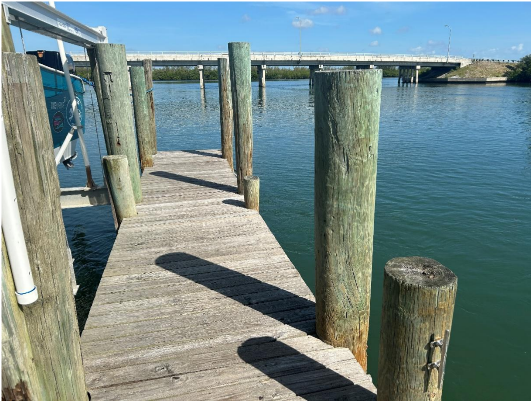
Photo 3: Northwest finger pier, cleats present for mooring, facing northwest.
