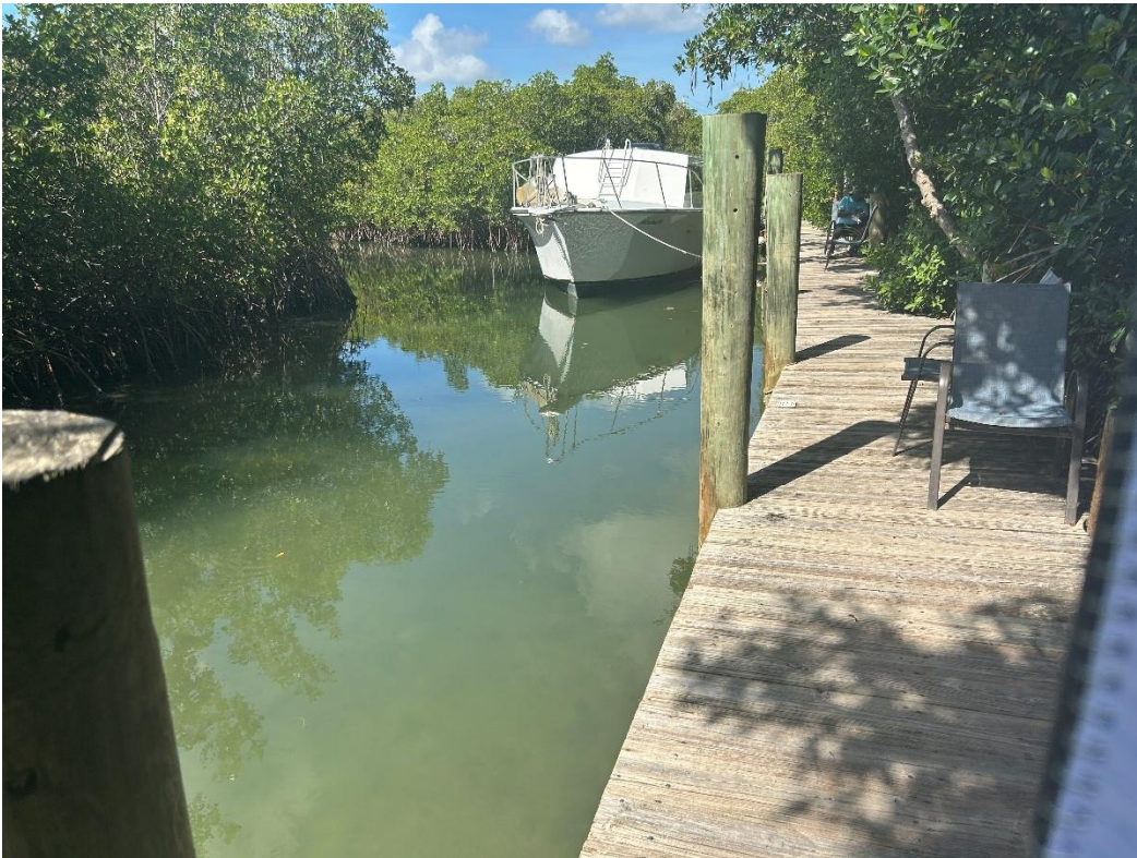
Photo 16: Southern dock, facing southwest.
