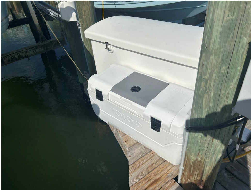
Photo 8: Small finger pier, used for deck boxes, facing southwest.
