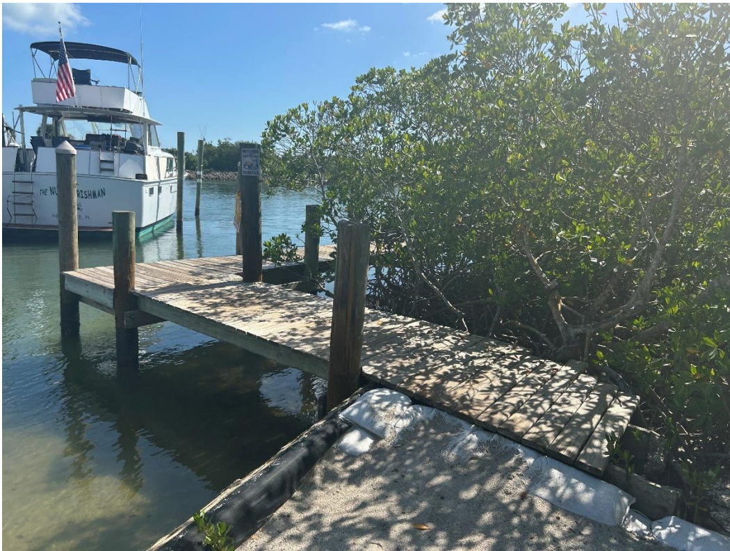
Photo 13: Eastern dock, over deeded submerged lands, facing east.
