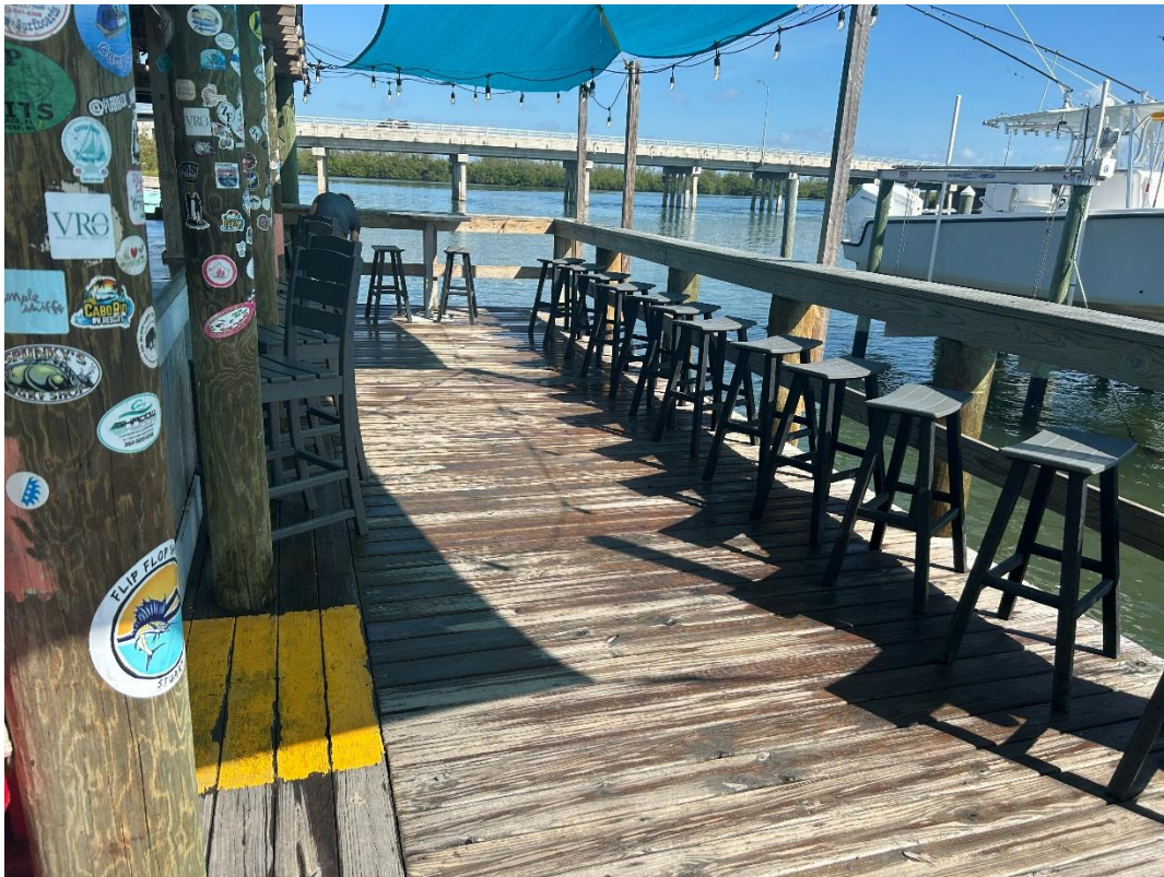
Photo 2: Overwater roofed structure and decking at beginning of dock facility, facing north.
