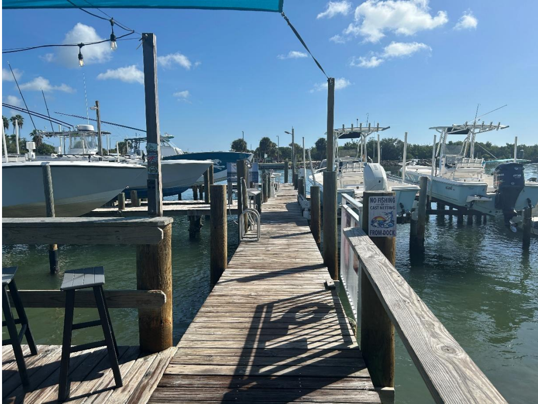
Photo 1: Dock facility overview, facing northeast.
