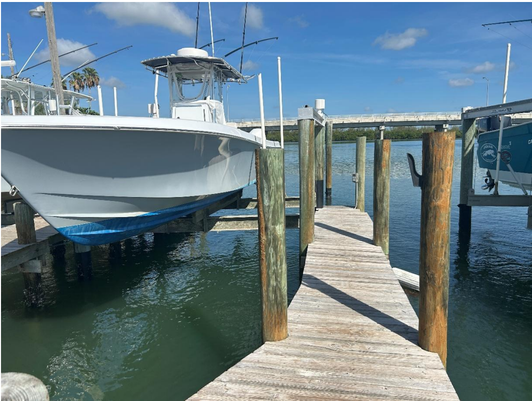
Photo 4: Middle northwestern finger pier, facing northwest.
