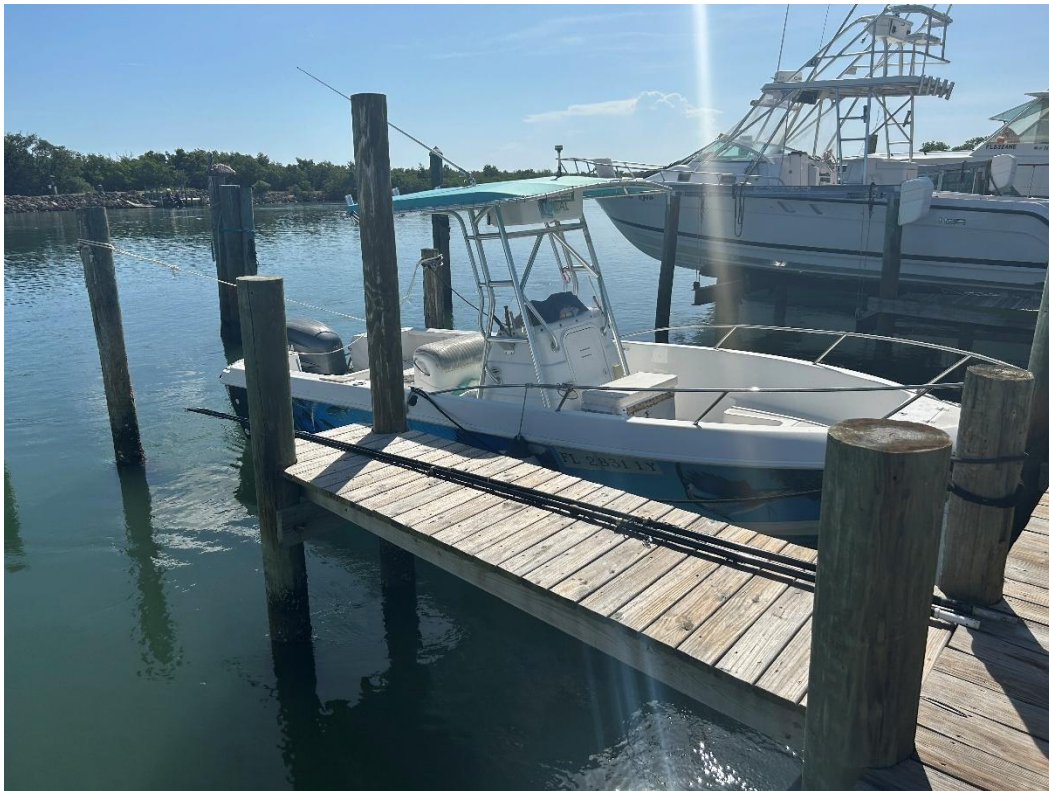
Photo 10: Finger pier, southeastern portion of main dock, facing northeast.
