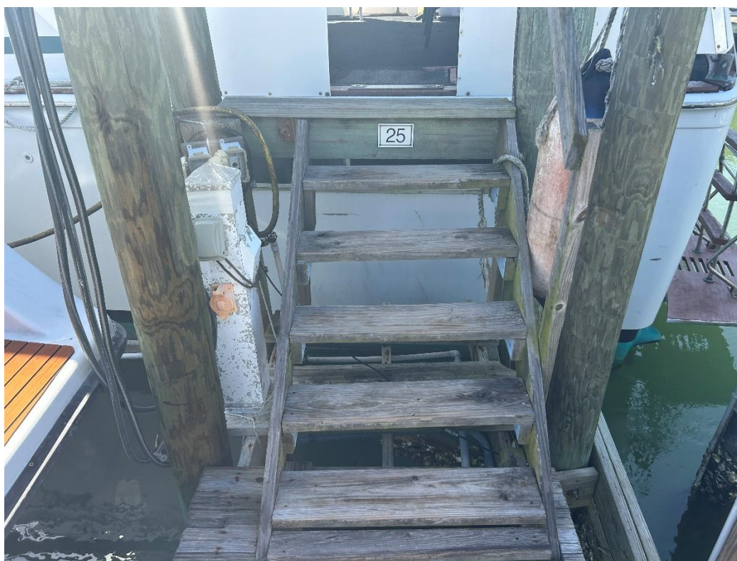
Photo 12: Terminal end of southeastern portion of main dock, facing southeast.
